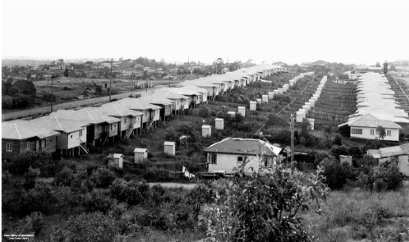
View from above of rows of timber houses with outhouses built by the Queensland Housing Commission, funded by the Commonwealth Bank, in Norman Park, Brisbane, Australia around 1950. Photo: Wikipedia
