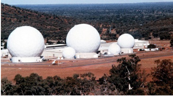
The Joint Defence Facility Pine Gap, in the Northern Territory, is used by the United States to collect intelligence and guide military strikes, including the Israeli strikes that are currently killing thousands of civilians in Gaza. Photo: AFP
