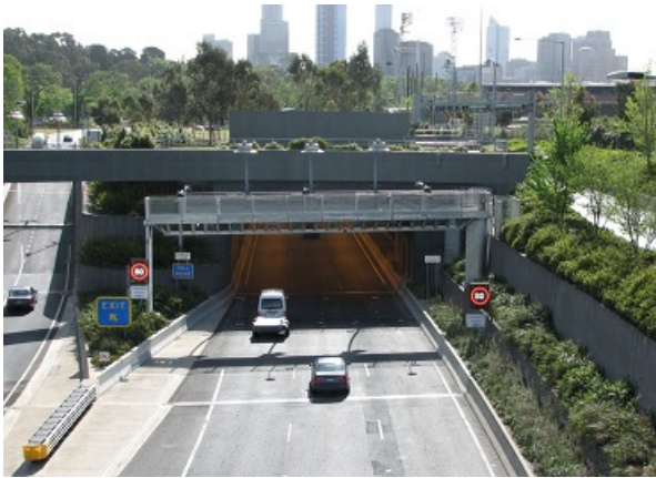
The Domain Tunnel on Citylink, Melbourne's major tollway owned by Transurban, which is one of the private infrastructure companies wanting a bailout from the government. If the infrastructure was public, there would be no need for bailouts. Photo: Wikipedia
