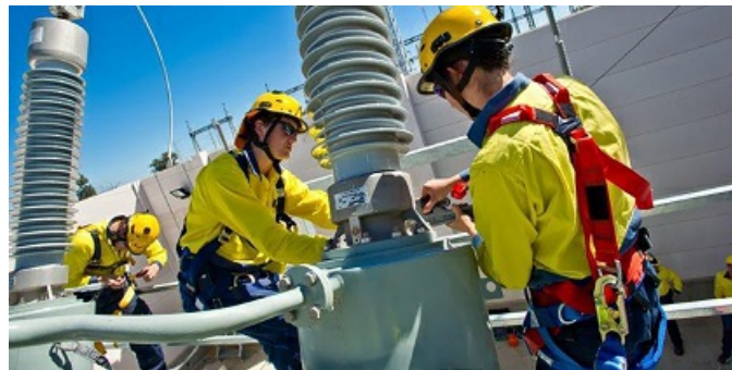
TransGrid servicing electricity substation. Photo: LinkedIn/TransGrid
