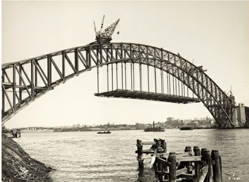
The Sydney Harbour Bridge, which required 52,800 tonnes of steel, under construction. Photo: Wikimedia Commons
