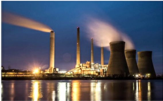
Could nuclear power plants help offset our aging coal generators?
