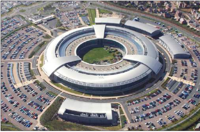
GCHQ's headquarters, a.k.a. "The Doughnut", in Cheltenham, England. US National Security Agency (NSA) whistleblower Edward Snowden proved in 2013 that GCHQ can and does monitor all UK phone and internet traffic; and former NSA Technical Director William Binney testified to the UK Parliament in 2016 that GCHQ unquestionably had the capacity to monitor all 3,000-odd individuals on MI5's watchlist in real time. Between this and MI5's own surveillance, it is not possible that so many known extremists could simply "slip through the net". Photo: Wikipedia
