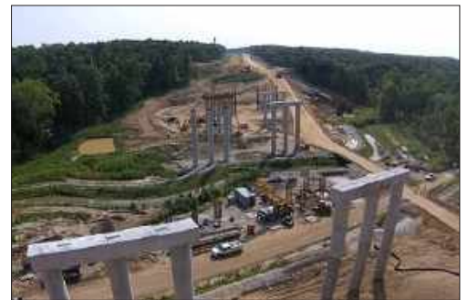
Construction of the I-69 tollway in Indiana. Photo: YouTube
