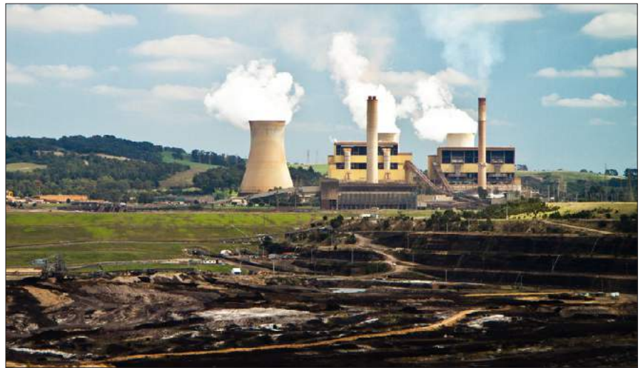
The Yallourn West Power Station in the Latrobe Valley was sold to a consortium including British company Powergen in 1996. Some 7,000 jobs were slashed in preparation for its sale, sending local job-losses to five times the national average for the early '90s. Photo: Wikipedia/Stephen Edmonds
