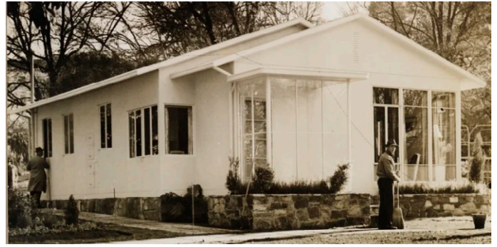
This prototype of a steel-frame prefabricated home, dubbed the Beaufort, was built in 1946 by repurposing wartime manufacturing plants used to build the Beaufort war-planes. Photo: State Library of NSW
