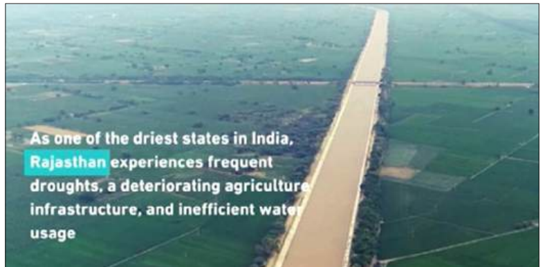
An NDB project: the Rajasthan Water Sector Restructuring Project in India—under construction, and completed canal. Photos: Screenshot/ndb.int
