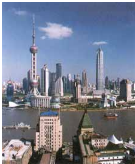
View of Pudong New Area of Shanghai from across the river. The load of the new buildings on the saturated sediments, together with groundwater pumping, is leading to subsidence of the area by about 3 cm. each year. It has been reported that 46 cities in China are sinking, due to settlement under load and excessive pumping of groundwater.
