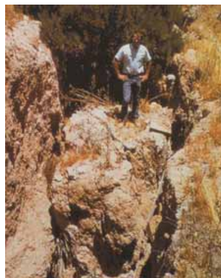
Subsidence related earth fissure due to groundwater extraction in Arizona. Fissures are causing very serious damage in several irrigation areas in the state. The Arizona Geological Survey maintains a Centre for Land Subsidence and Earth Fissure Information. Information papers are available on the internet. (Source: Govt Arizona)
