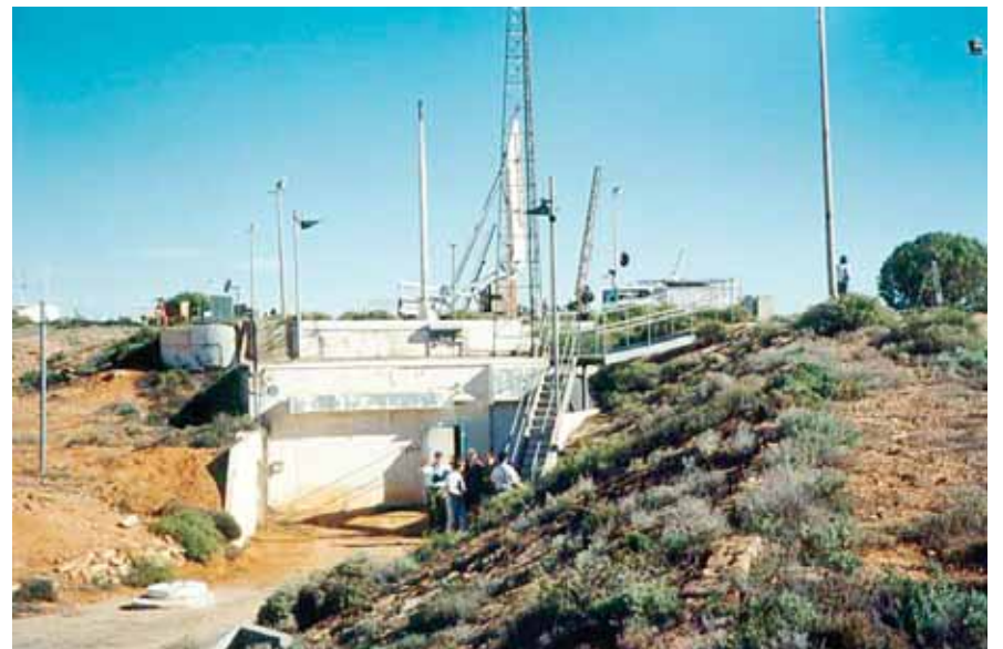
Above Left: The blockhouse at the Woomera test range, where Australia first joined the space age. Engineers and launch directors took shelter inside the blockhouse during a test or launch, and watched the pad from a periscope inside. Photo: Australian Space Research Institute
